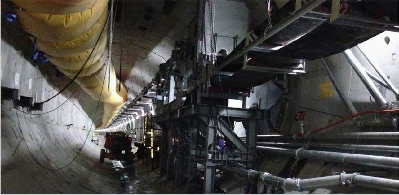
Figure 2: The ventilation bag (top left) carried fresh air from the surface to the tunnel boring machine.
